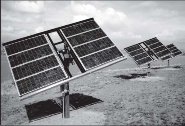
Figure 2. A 1-kilowatt PV deployment provides water pumping (Photo courtesy NREL/PIX.)
