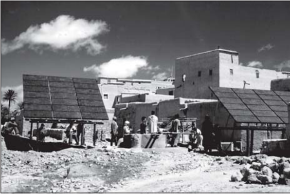
Figure 3. A 2-kilowatt PV deployment provides village electricity. (Photo courtesy SEIA.)
