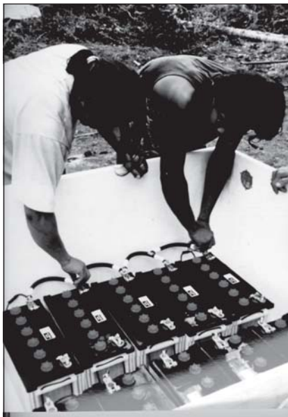
Figure 6. A bank of batteries in an acid-proof container stores energy from a 1-kW PV system. (Photo by S. Thornton, courtesy NREL/PIX.)
