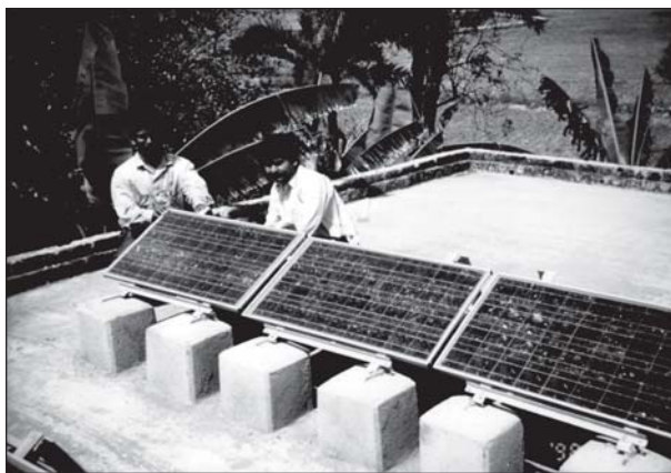
Figure 8. Modules at a clinic in Sundarbans, West Bengal, India, are fixed to a frame and anchored in concrete. (Photo by J. Welch, courtesy NREL/PIX.)
